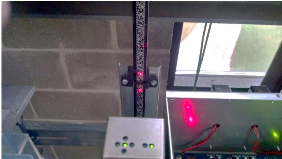
Figure 2-21: APS Selector Alignment Spotlights
