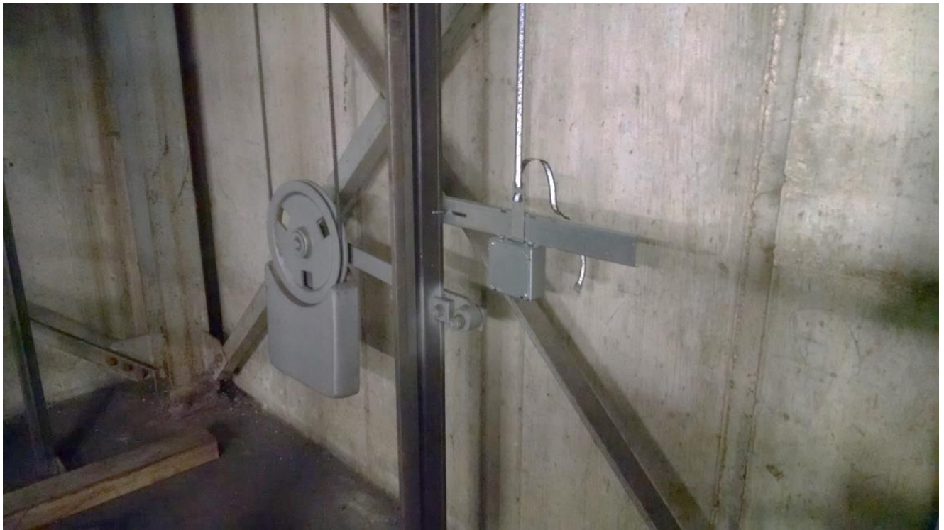
Figure 2-8: Encoded Tape Mounting – Bottom Bracket
