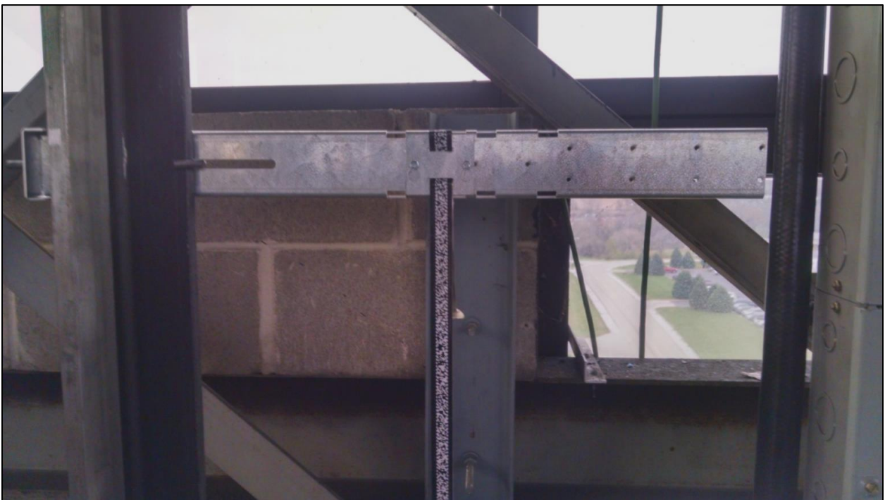
Figure 2-1: Encoded Tape Mounting – Top Bracket
